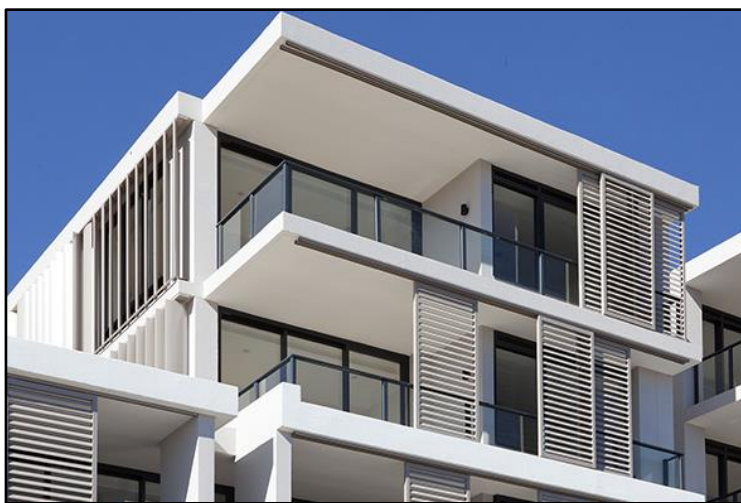
Figure 13: Privacy treatment integrated in the building design to mitigate privacy impacts (Source: Google)
