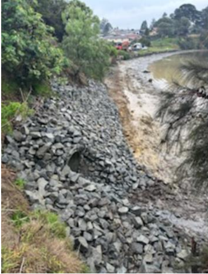
Figure 2: Image of repaired stormwater outlet at Casuarina (supplied by GCC; 22/08/24).
