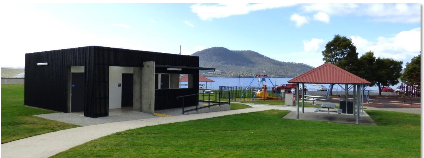
Below: Montrose Bay Foreshore toilet block
