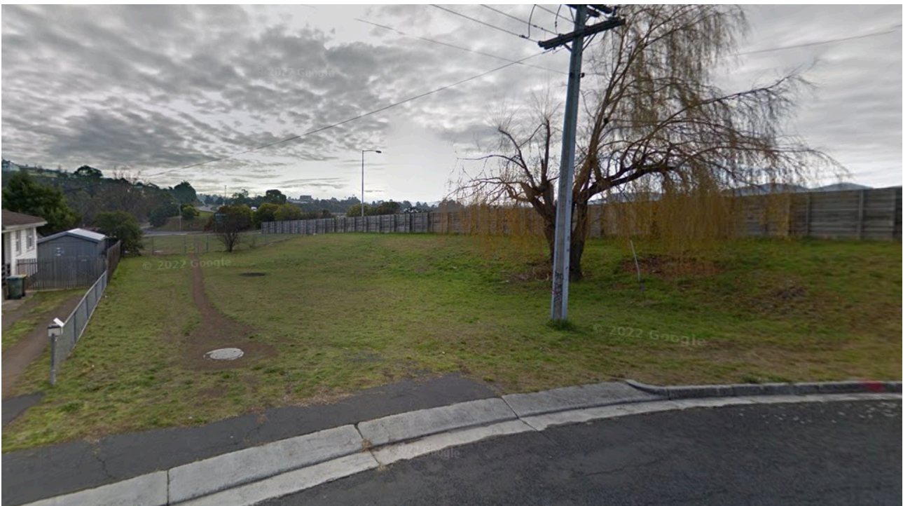
FIGURE 3.2: SITE AND EXISTING BARRIER - LOOKING NORTH
