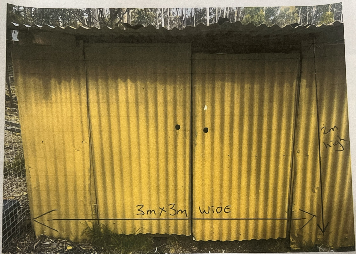
Additional Storage Shed 2 Springdale Road Collinsvale
