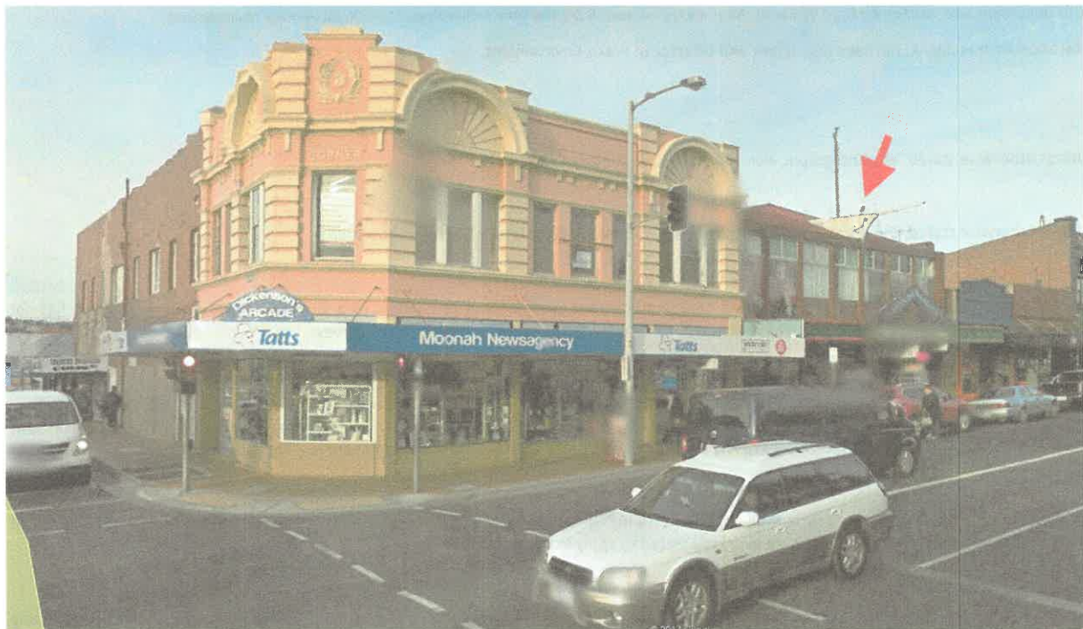
Figure 1.1 – Overview of 105-111 Main Road, Moonah, the red arrow depicting the windjammer. Adapted from Google Streetview .
