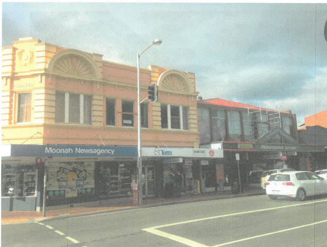
Figure 4.1 – Overview of the Main Road frontage of the Baker's Corner and Dickenson's Arcade buildings.
